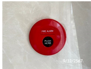
Fire Alarm Manual Station
