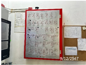
Graphic Annunciator Fire Alarm System
